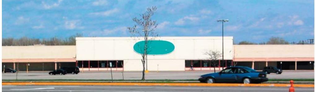
Figure 10. Vacant retail along Transit Road.
