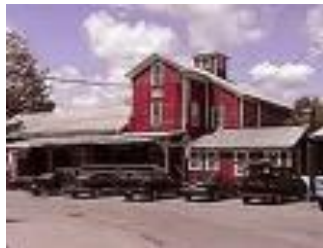
(Williamsville Water Mill)
