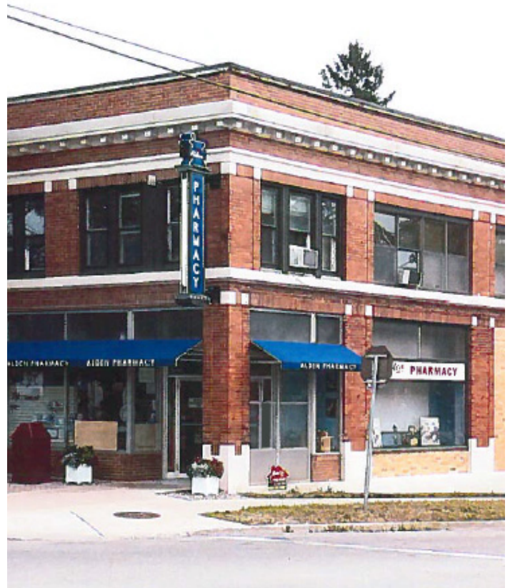
Recent façade improvements to the Alden Pharmacy (Source: Erie County)
