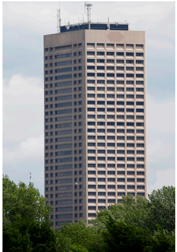
The redeveloped Seneca One Tower will act as a downtown anchor with a mix of commercial, residential, and retail space.
