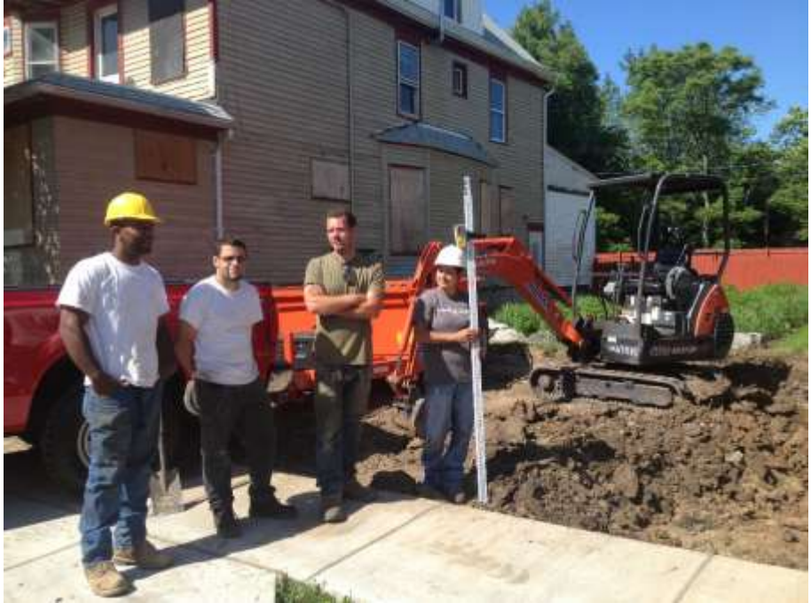
PUSH Blue's Green Infrastructure Team on site
