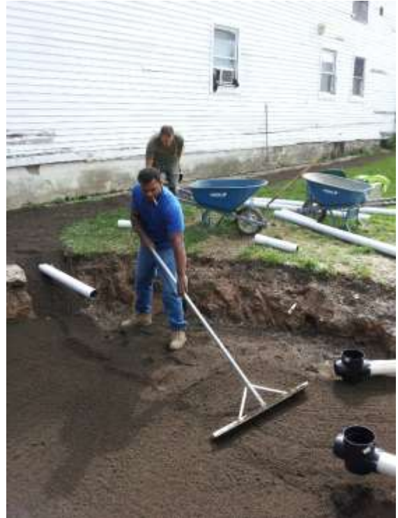
PUSH Blue crew working on green infrastructure in Buffalo’s west side
