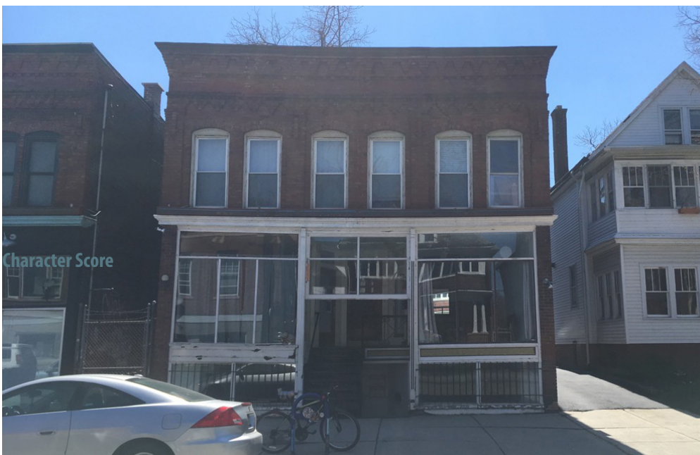
Building on Potomac avenue threatened with demolition for the arbor + REverie Project. Photo by Andrew Varuzzo
