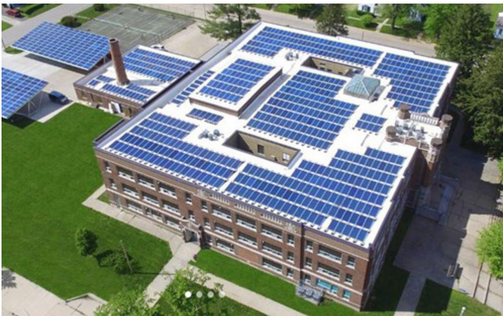
Case 1: The former Fort Madison, IA middle school was recently converted into 38 apartments at a cost of $4.6 million. The rehabilitated building features a 300kW solar array that offsets residents' electricity costs by up to 100%. 11
