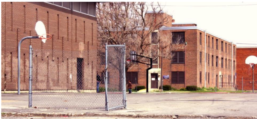
Figure 10: Lanigan Field House
