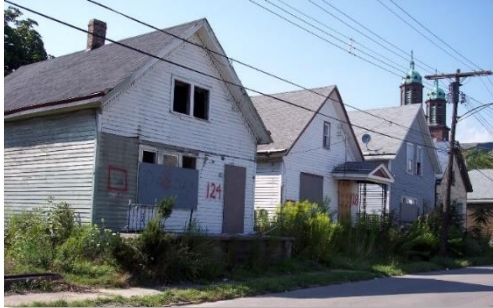
Figure 11 Unoccupied residential homes marked for demolition on Sears Street. Digital Image. Wikimedia Commons. August 17, 2008. https://commons.wikimedia.org/wiki/File:East_buffalo_decay.JPG .
