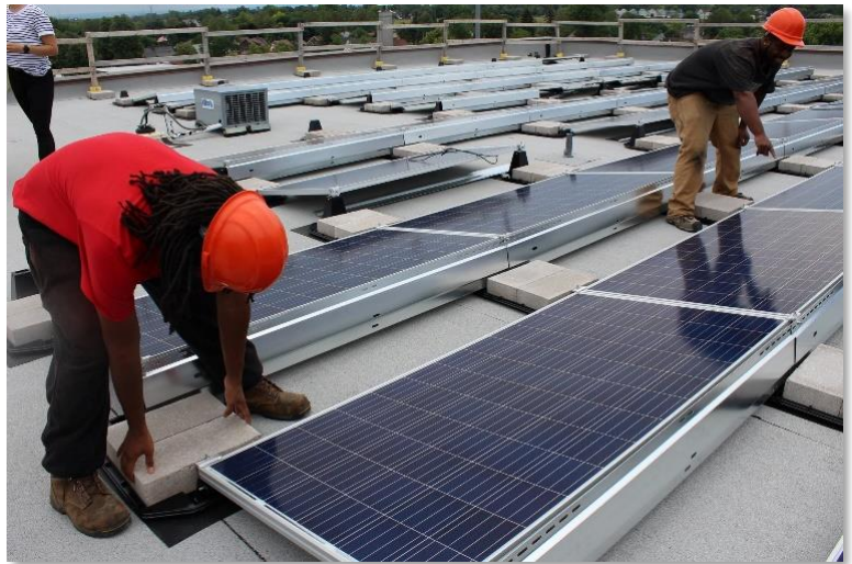
Figure 8 PUSH Buffalo. Hiring hall, solar install. Digital Image. Facebook. July 11, 2017. https://www.facebook.com/push.buffalo/photos/a.846721715504799.1073741835.375021042674871/846722635504707/?type=3&theater
