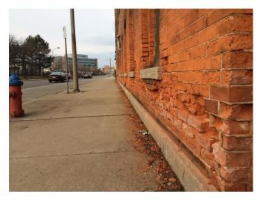
A cocktail of traffic pollutants including rock salt and reactive chemicals like nitrogen oxides (NOX) is causing the brick on this privately owned building on Elm Street in Buffalo to decompose prematurely.
