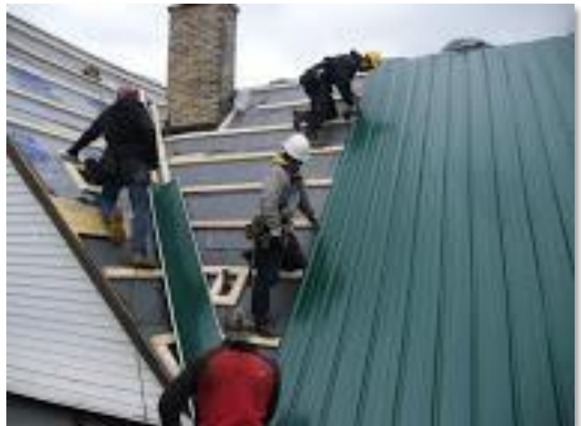
Figure 12 PUSH Buffalo. Roof Repair. Digital Image. Facebook. April 11, 2016. https://www.facebook.com/PUSHGreenWNY/photos/a.350148401703733.102336.284211014964139/1106236206094945/?type=3&theater .
