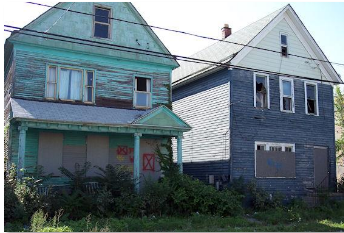
Figure 3 Two unoccupied residential homes in Buffalo, NY. Digital Image. Wikimedia. Accessed November 10, 2017. https://commons.wikimedia.org/wiki/File:Buffalodecay1.jpg .
