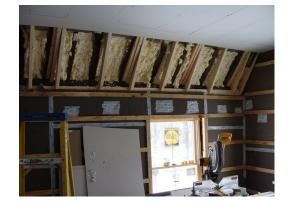
Zero house not only to use clean energy, but to use energy more efficiently. With this concept in mind, PUSH Buffalo created a "thermal envelope", insulating the house with three different types of insulation. They first installed rigid foam board over the studs of the house; then they had dense pack cellulose blown into the spaces between the foam board and the studs. Finally, they used spray foam insulation was to insulate any small cracks that might allow energy to escape.
