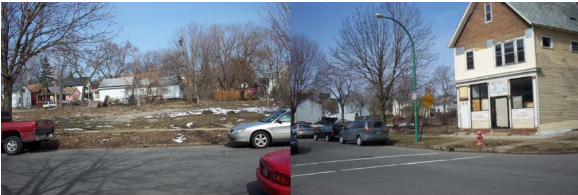
Figure 1: Unkept Vacant Lots and Abandoned Structures Fronting Futures Academy 2
